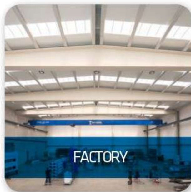
Custom manufacturing of water treatment facilities
