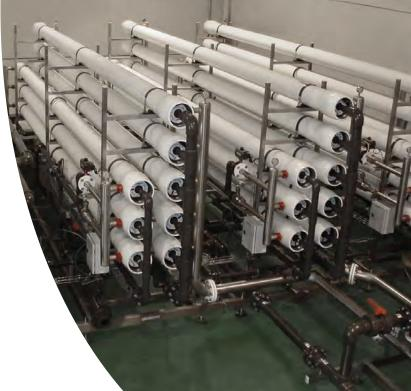
Reverse osmosis is a membrane technology that removes salinity from water. It is based on a diffusion process through a semipermeable membrane that facilitates the passage of dissolved gases and molecules without electrostatic charge of low molecular weight.
