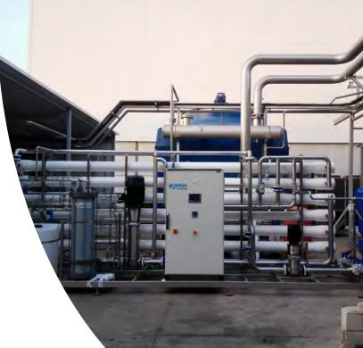
Treatment for the elimination of dissolved ions in water through ion exchange resins that are reactivated by the use of regenerants.
