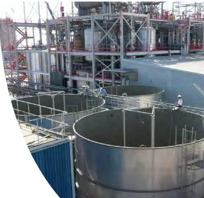
In those sectors where the biodegradable pollutant load is very high, anaerobic microorganisms are used. Biogas (mainly CH4 and CO2) and a small fraction of sludge are obtained as by-products. On occasions, the effluent obtained does not meet the minimum quality requirements and therefore requires additional refining treatment.
